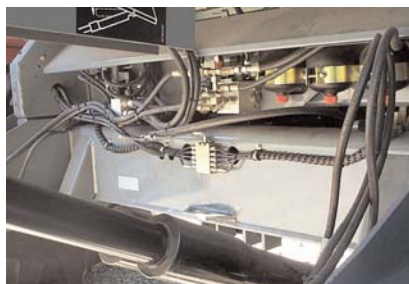
Progressive feeders on the front axle for supply of lube points on leveler (balance).
